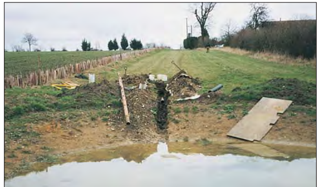
An agricultural field drain is intercepted and brought to the pond edge with pipework as a water supply
